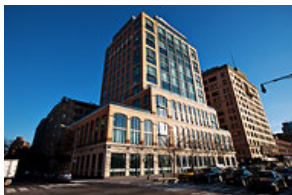
Benjamin Norman for The New York Times Superior Ink, 400 West 12th Street, is moving its mechanical systems above ground, and mulling the purchase of a generator.
